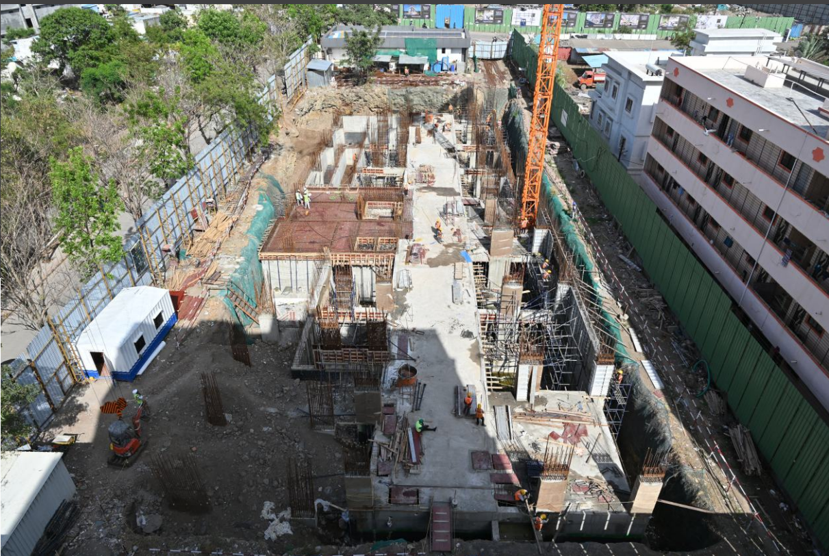
1 st slab RCC Work in progress.
